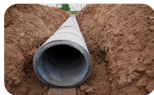
SEWAGE PIPE LINE
